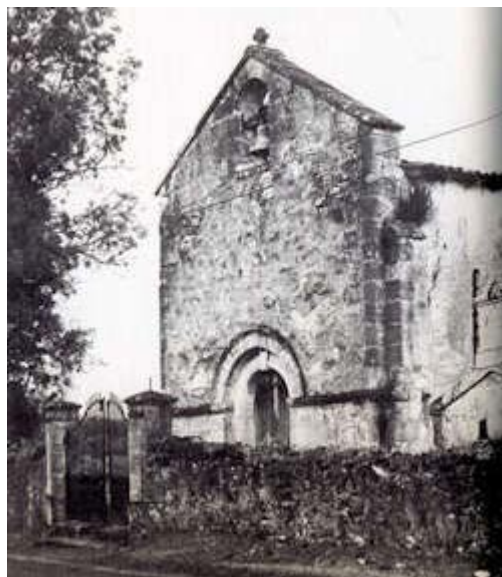
Lugeras, facade occidentale - Image M. Miguet
